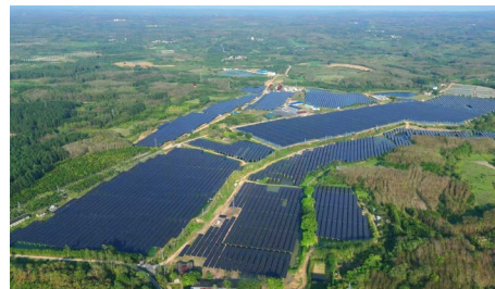
Ding'an Flexible Mounting Project in Hainan
