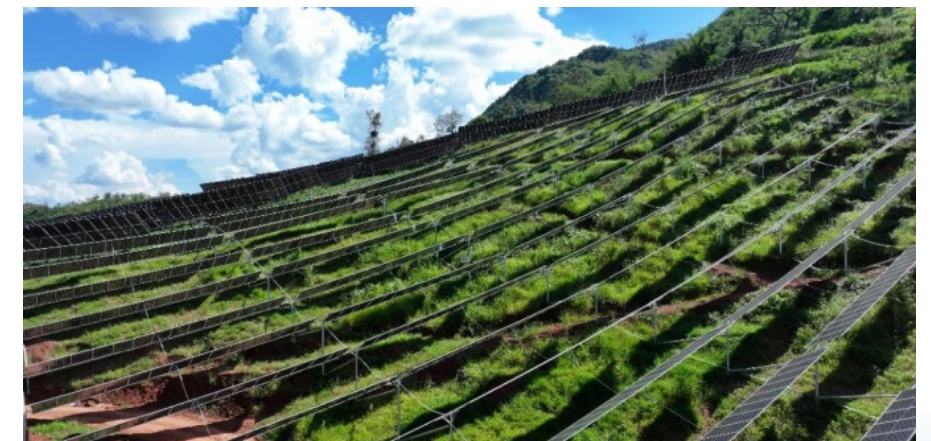
Yimen Flexible Mounting Project in Yunnan
